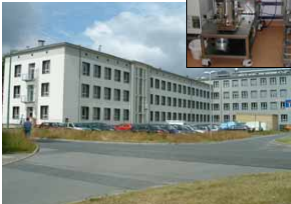
Office and lab building 8a Microbiological and radiochemical labs, Divisions Biogeochemistry, Surface Processes, Biophysics
