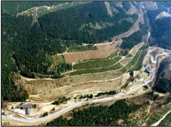
Uranium mining waste pile “Haberland” nearby Johann- georgenstadt, Saxony
